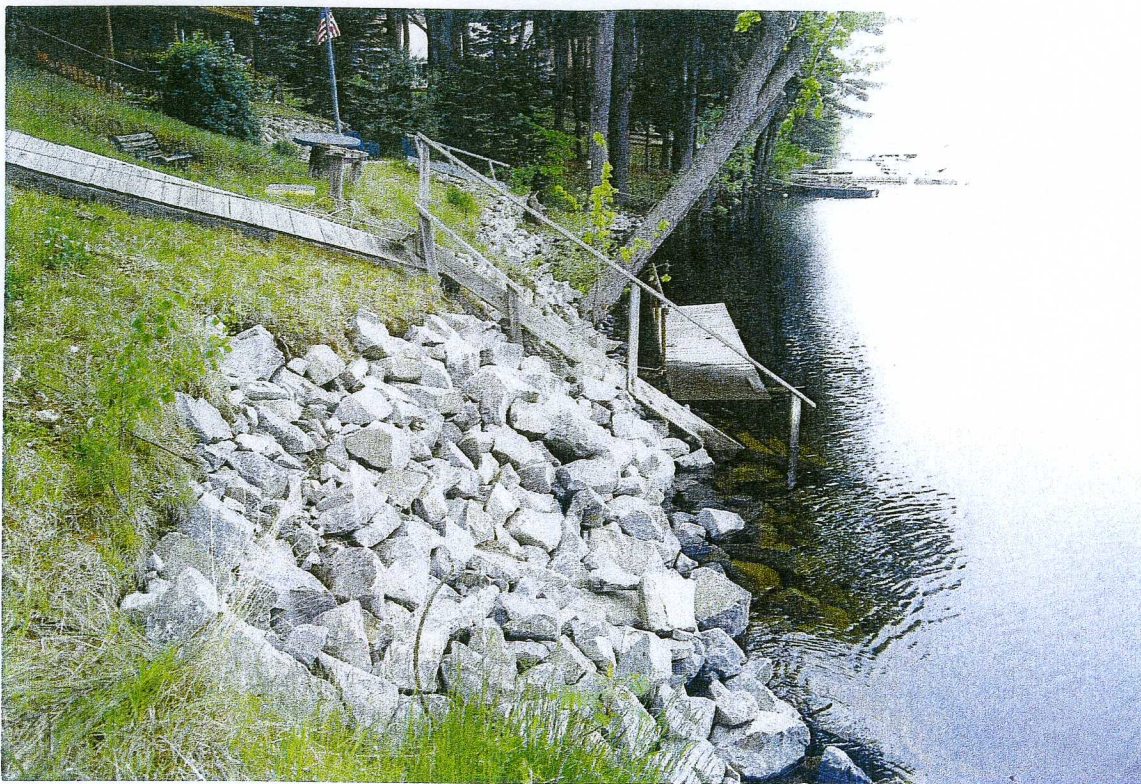
Photo 8. View northeast of freshly-deposited rip-rap in an eroded area. The Regulating District routinely repairs shoreline erosion at Great Sacandaga Lake.
