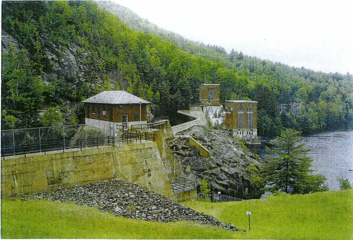
Photo 4. View northeast of facilities at the Conklingville Dam showing from left to right: the control house, the power canal, the spillway, the E. J. West hydroelectric plant, and Stewart's Bridge Reservoir.
