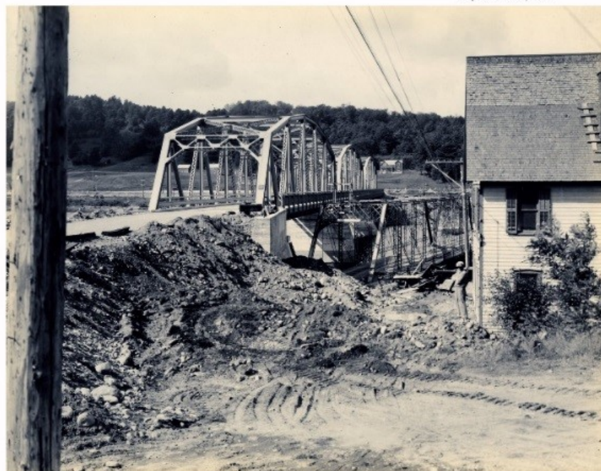
Northville Bridge under construction in 1929, replacing old bridge in center before reservoir began operation.
