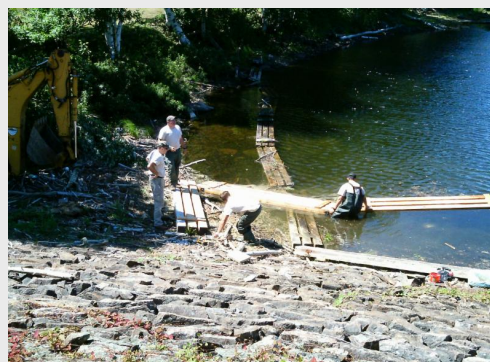
Summer interns work on repairing the log boom at the Indian Lake Dam.
